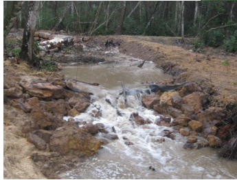
Natural Stream Restoration Workshops
